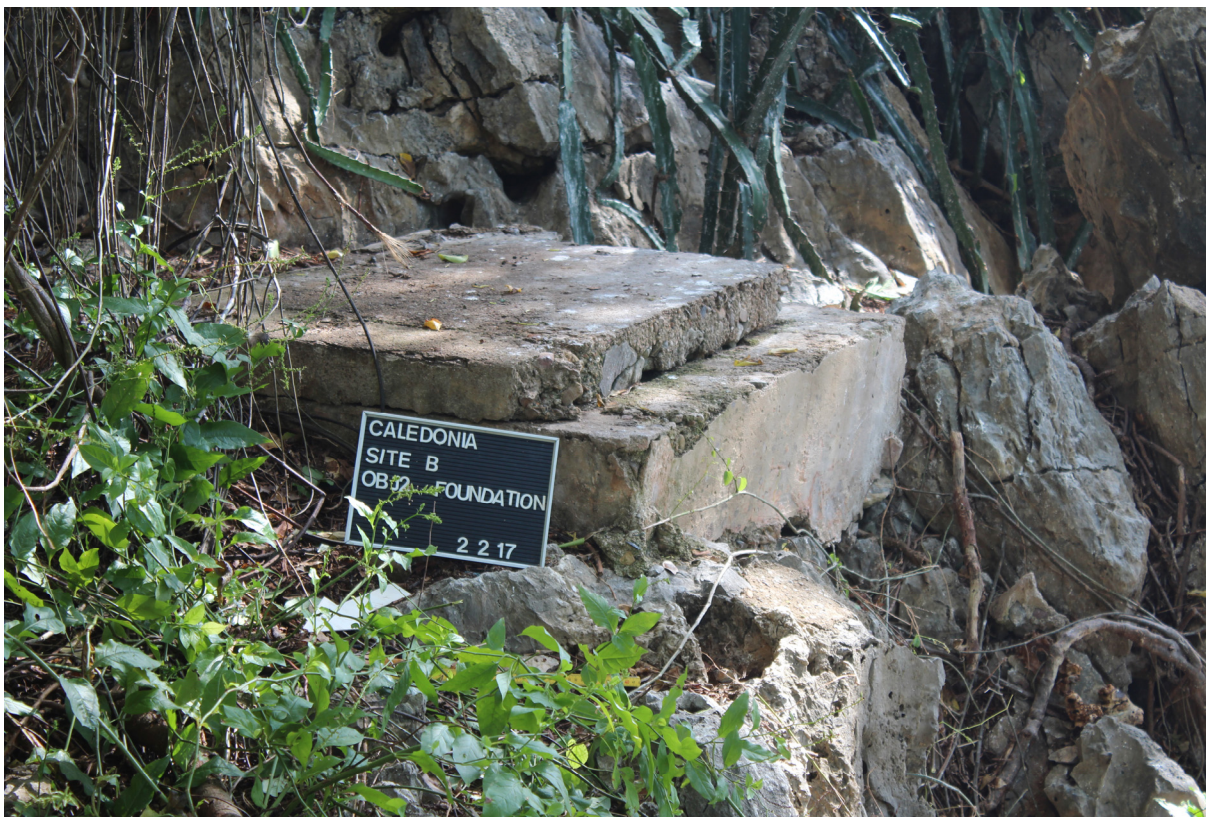
Figure 11: Eastern foundation as seen from the west
