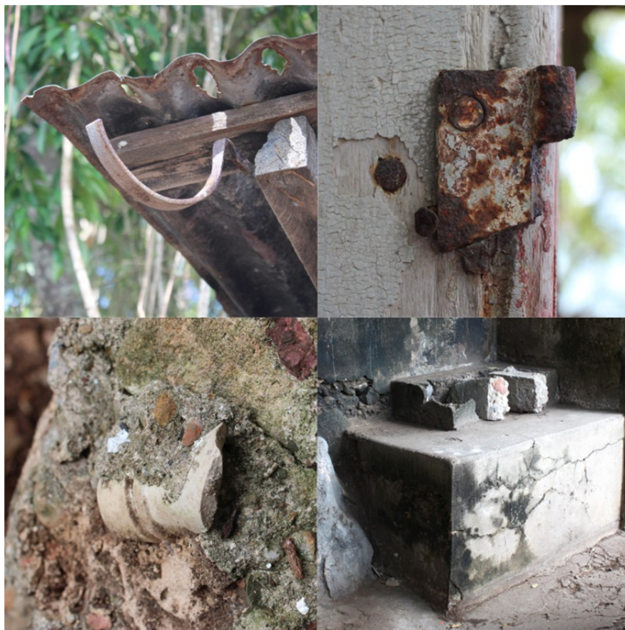
Figure 6: Details of kitchen building. a) hook for rain pipe, b) hinge for window in north-western wall, c) walled-in fragment of bottle in south-western wall, d) stove in eastern corner
